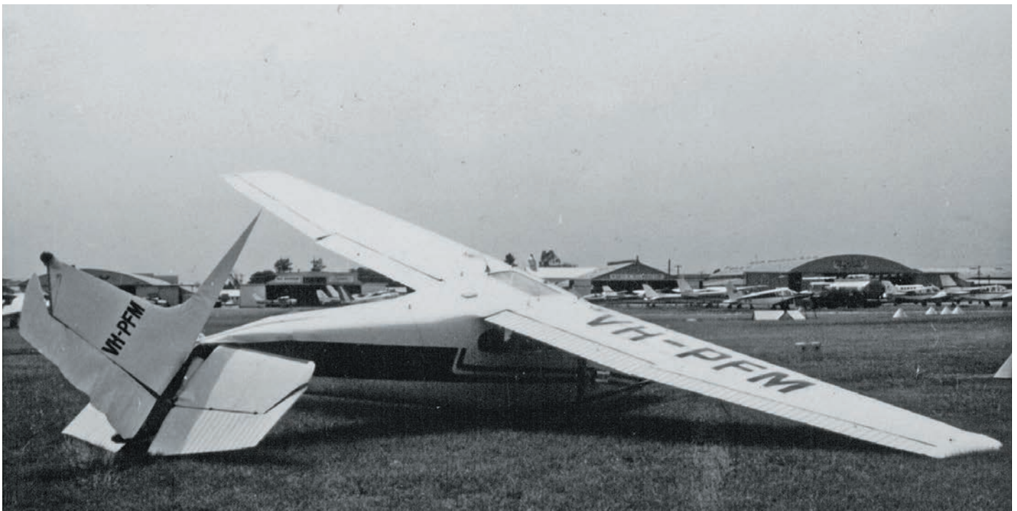
The Cessna despite being tied down was significantly damaged by the 141km/hr winds that hit Archerfield during a storm in 1980.
